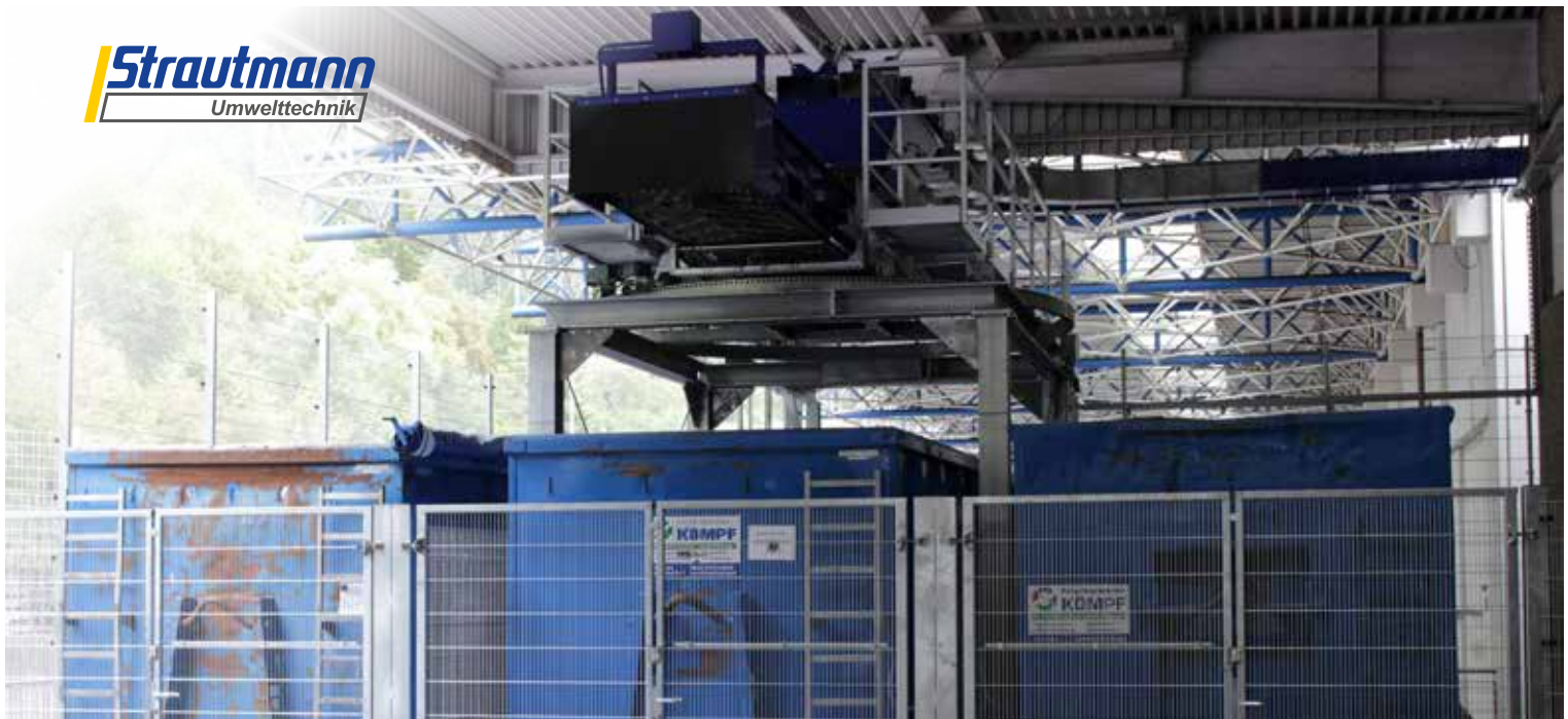
Automatic briquette distribution on three containers
